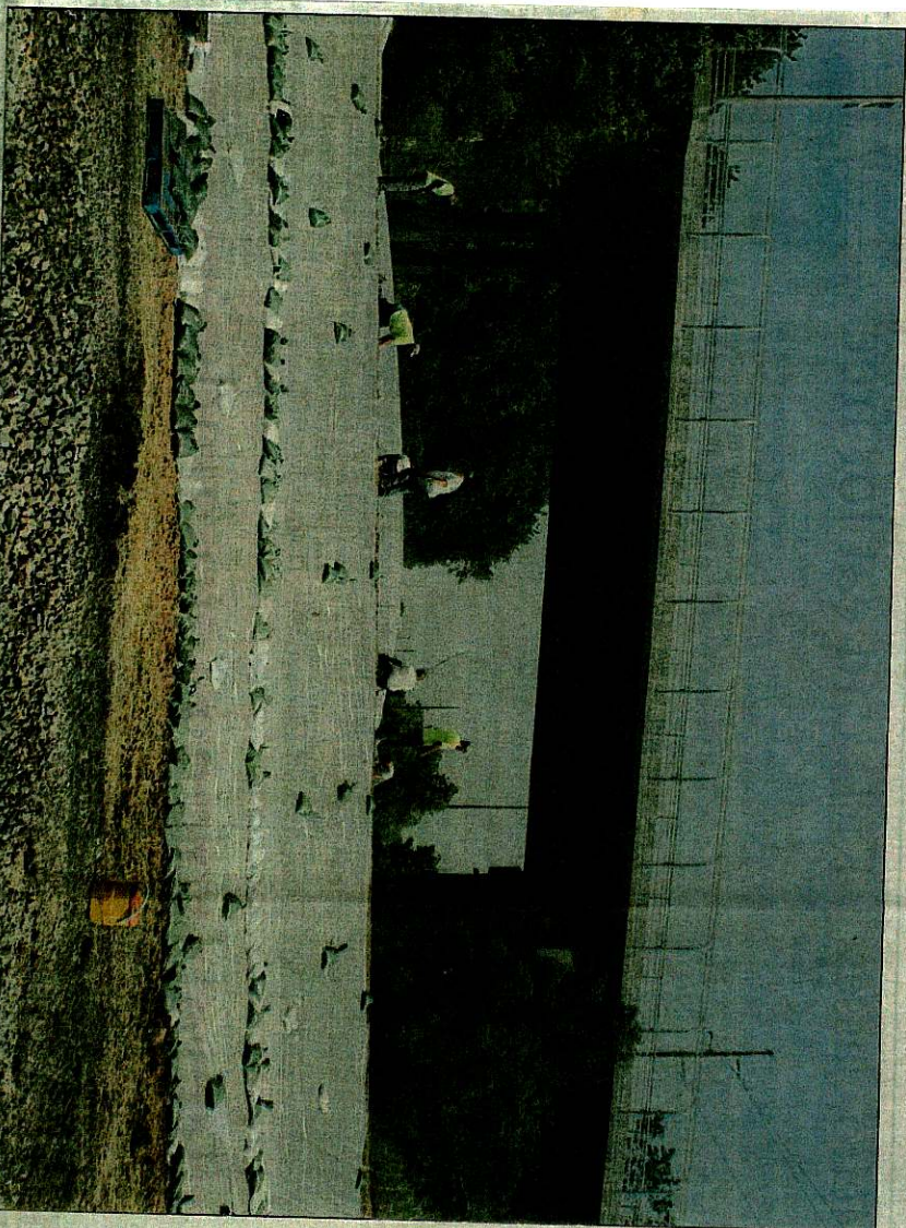
Submitted by Phil Davidson, City of Bellevue Workers with the Popple-Missouri River Natural Resources District put the last sheet of plastic over the berm under the highway near Haworth Park on Tuesday. Once the plastic is down, they could put the rest of the 5,000 sandbags on top. The berm is to protect Harlan Lewis Road and areas to the southwest of Haworth Park. In addition to Haworth Loop Hiking/Biking Trail, remains closed. The trail runs south from Haworth Park along the Missouri River to the confluence with the Popple Creek, then northwest to Capetown Road near 13th Street.
